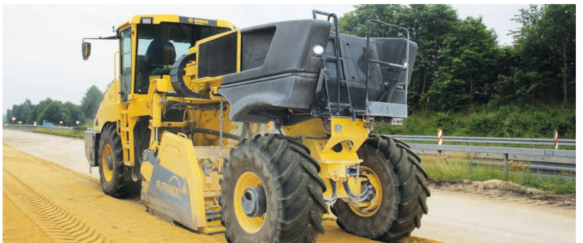
Milling a hydraulically bound base course.
