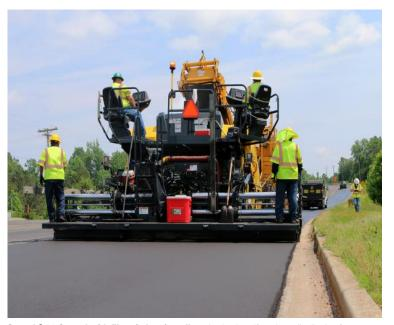
**Stretch® 20 Screed with Electric heating** offers absolutely uniform heat distribution for a quality mat. The flexible paving width of 10- to 30-feet makes the CR 1030 W ideal for a variety of applications. Stretch® 20 Screed has wear-resistant, durable steel plates for long lifespan and reduced maintenance.
